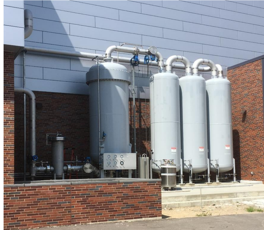
Final oil removal (outside, south side)
