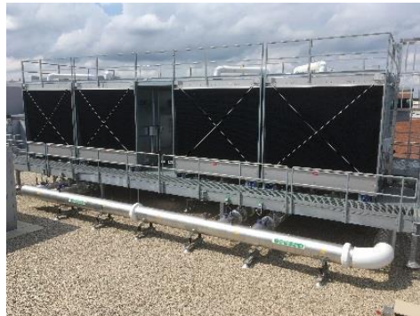
Cooling Tower Loop
