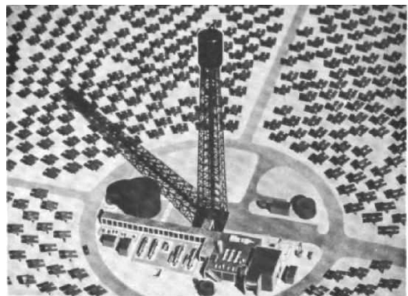
Figure 2-15. Model of 10-MW e Solar Thermal Central Receiver Pilot Plant
