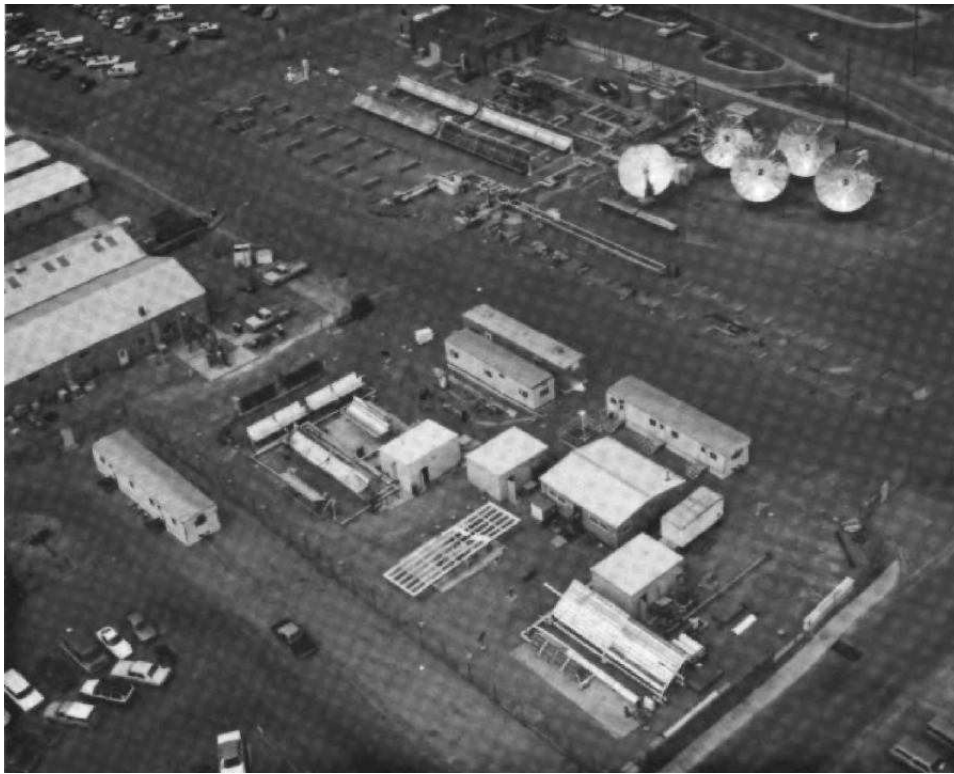
Figure 3-9. Midtemperature Solar System Test Facility
