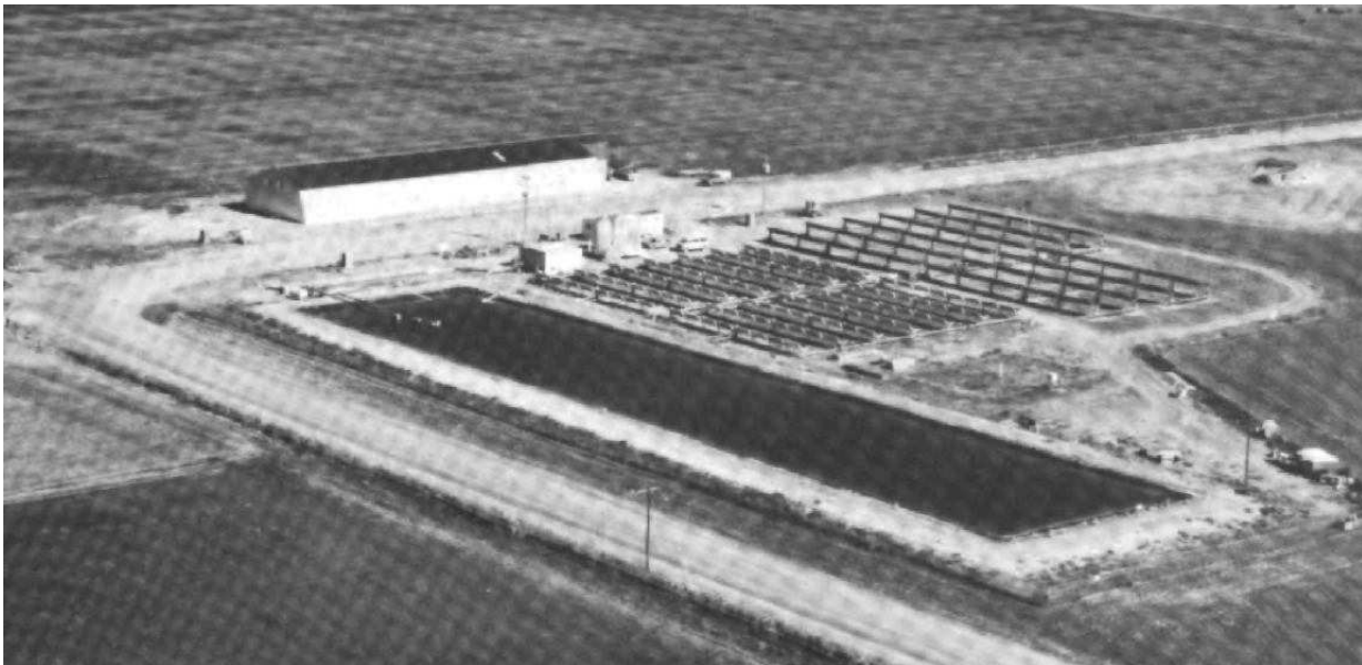
Figure 3-12. Shallow Well Irrigation, Willard, N.M.
