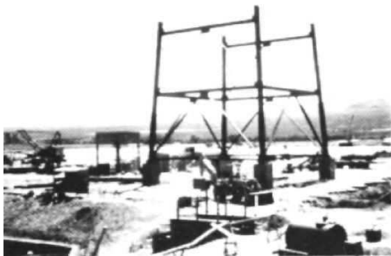
Figure 2-20. Ten-MW e Receiver Tower Under Construction
