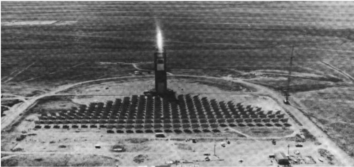
Figure 2-12. Central Receiver Test Facility
