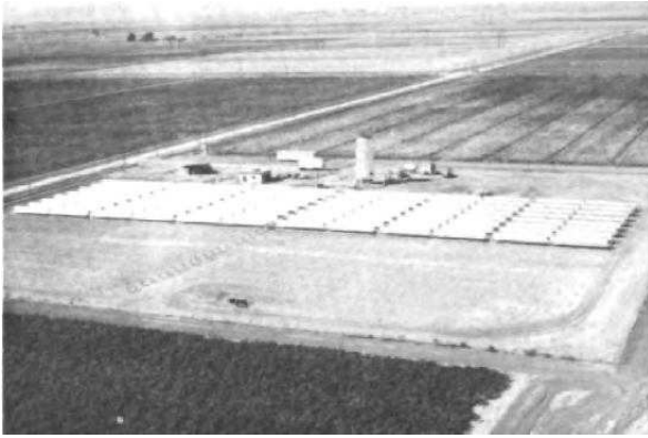
Figure 3-13. Deep-Well Irrigation, Coolidge, Ariz.
